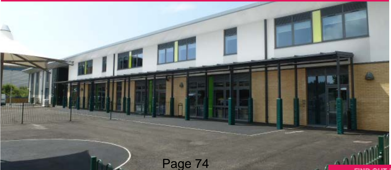
Recent new build primary school in Cardiff - Ysgol Glan Morfa
